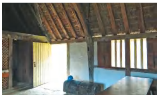
An interior shot showing door and window. The window has wooden mullions but no glass at this date, which shows how dark the interiors of these buildings were! Photograph courtesy of G. Grime, Weald & Downland Museum
